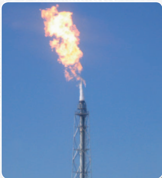
HCL Low Noise / High Efficiency Steam Assisted Flare
