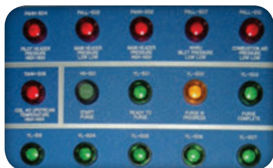
Control panel burner management system
